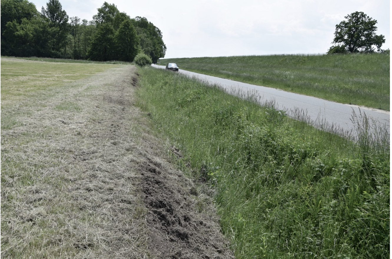
Flood embankments on the Bolko Island
