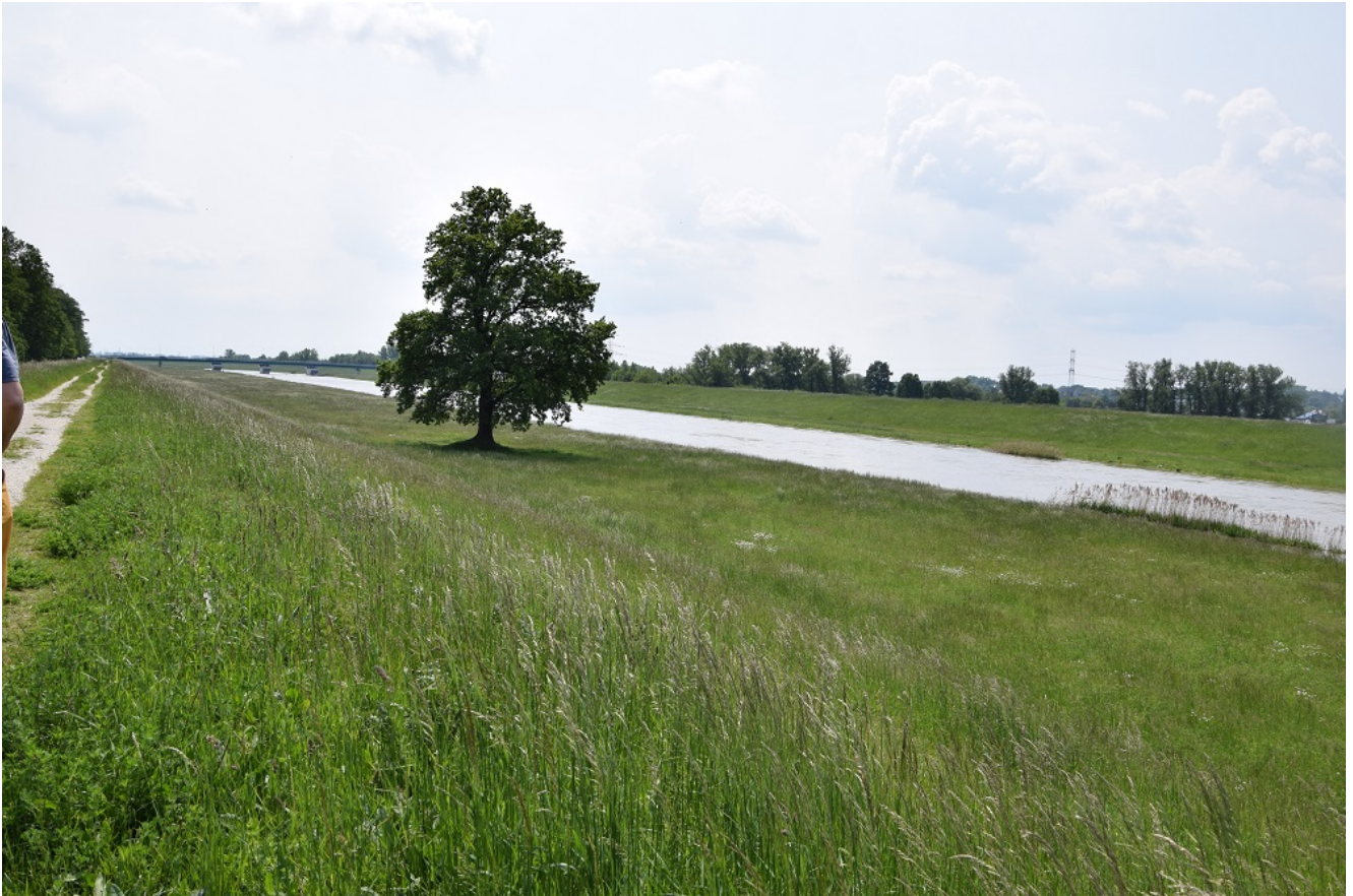
Flood embankments on the Bolko island
